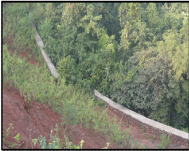
Photo – 2 & 3 – Showing Retaining Wall along with plantations at the toe of dump slopes
