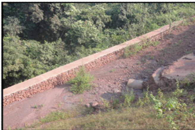
Photo 8– Check Weirs to check Run-off
